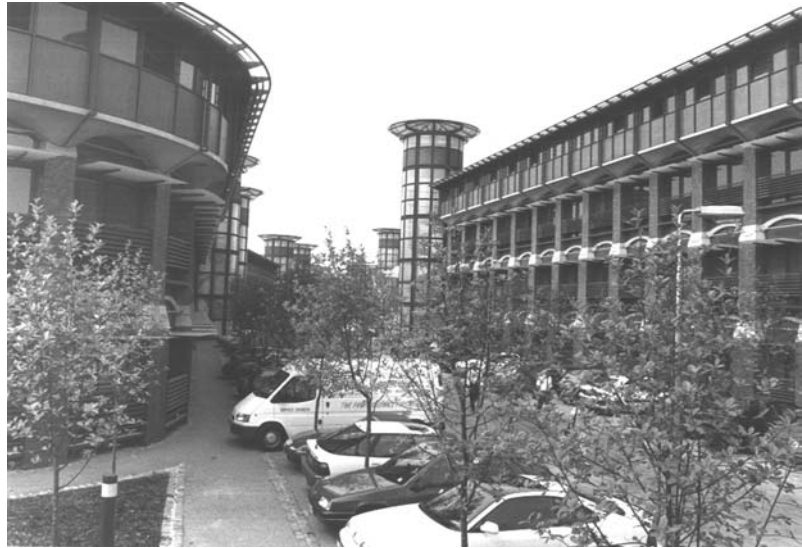
Figure 9.39 Inland Revenue Building, Nottingham
