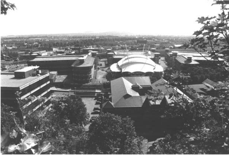
Figure 9.37 Inland Revenue Building, Nottingham
