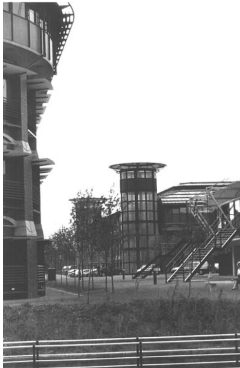
Figure 9.38 Inland Revenue Building, Nottingham
